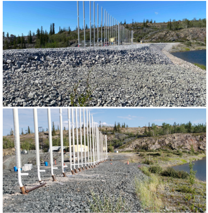
Photo 32: Dam 1 Crest Raise (before and after construction)
