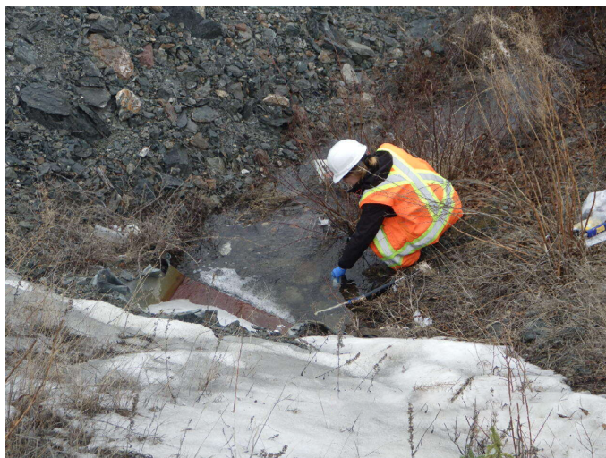
Photo 10: View of Surface Runoff on Site
