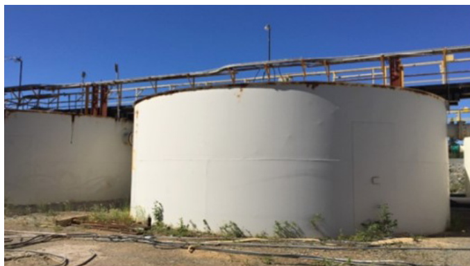
Photo 14: Giant Mine Old Effluent Treatment Plant
