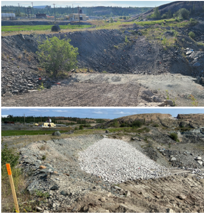
Photo 31: B2 Dam Slope Remediation (before and after construction)
