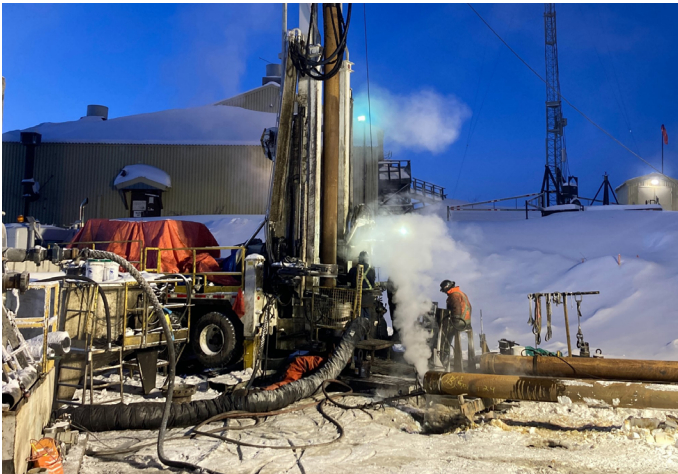
Photo 29: Drilling and Well into the Underground Left photo: drill rig on site for the new water intake for the water treatment plant Right photo: completed well
