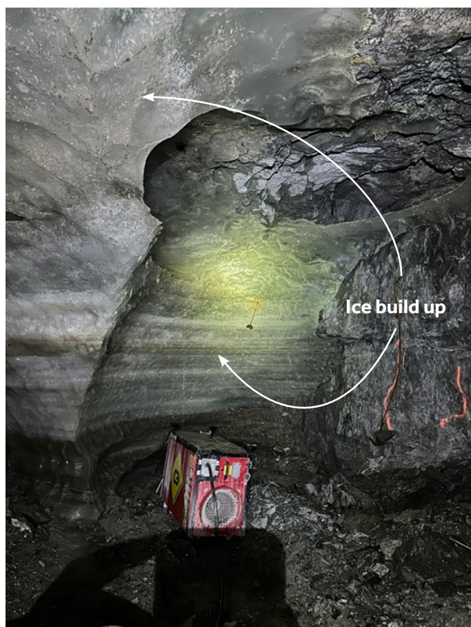
Photo 45: Ice Buildup Underground that Could Block Access to Areas for Remediation (heater was used to melt the ice)
